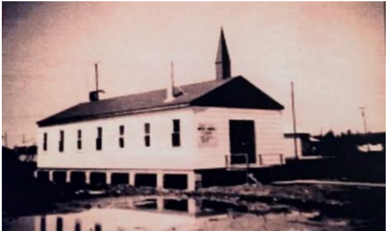
Original temporary building
