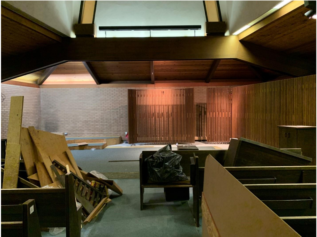
Mid-way through chancel renovation
